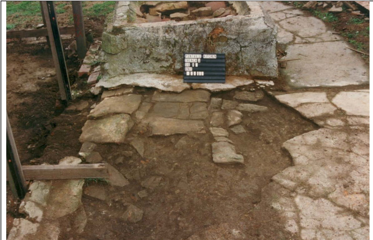
Photograph 51 Large blocks of stone, some rounded from wear, can be seen here below the thin mortar layer at the stone stand. A dilapidated spoon drain composed of concrete and brick can be seen between the path and the location of the kitchen wall, left.
