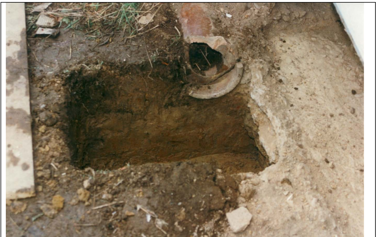
Photograph 58 Seen here is test pit in Trench 4 revealing a thin concrete footing, right, beneath the outer wall of the east verandah and a shallow trench for a ceramic storm water pipe. The clay beneath the pipe appears to be undisturbed.
