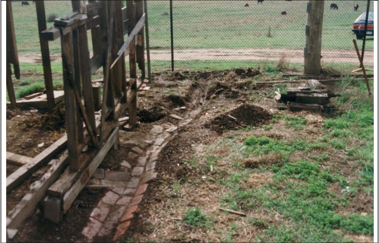
Photograph 55 Seen here is the spoon drain that collected waste from the wash room of the kitchen
