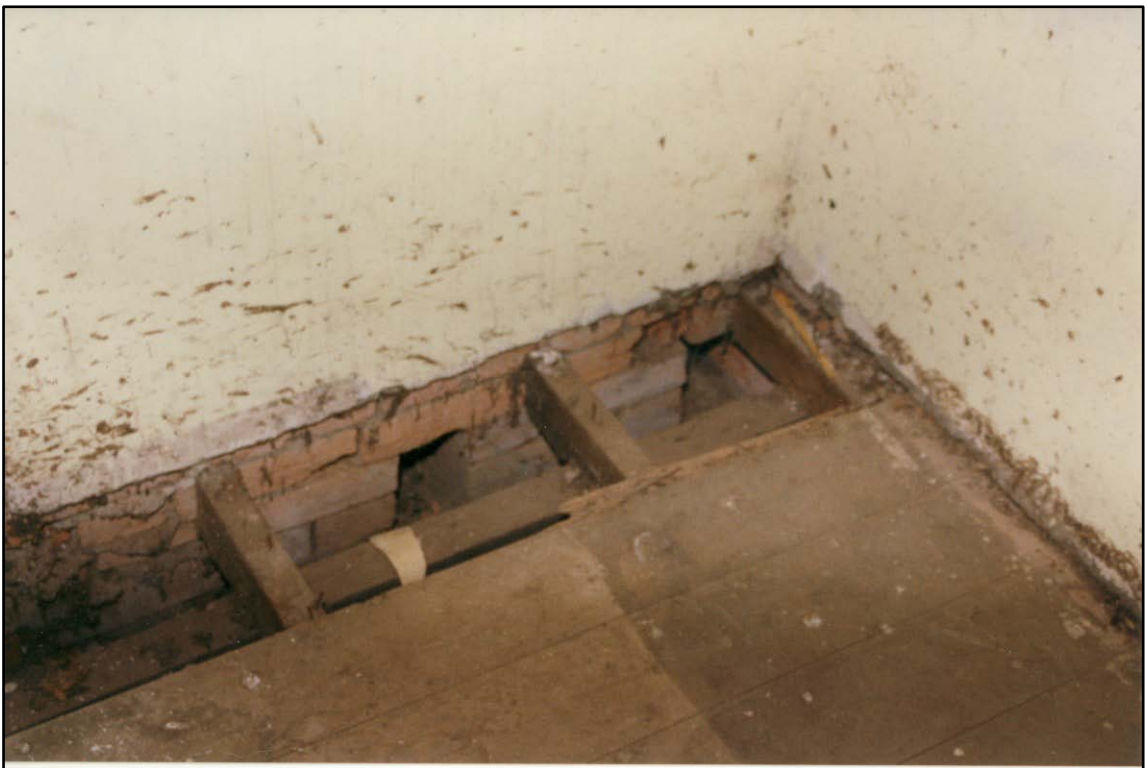
Photograph 13 Sub-floor opening in north room showing joist insert holes in walls and underfloor vents.
