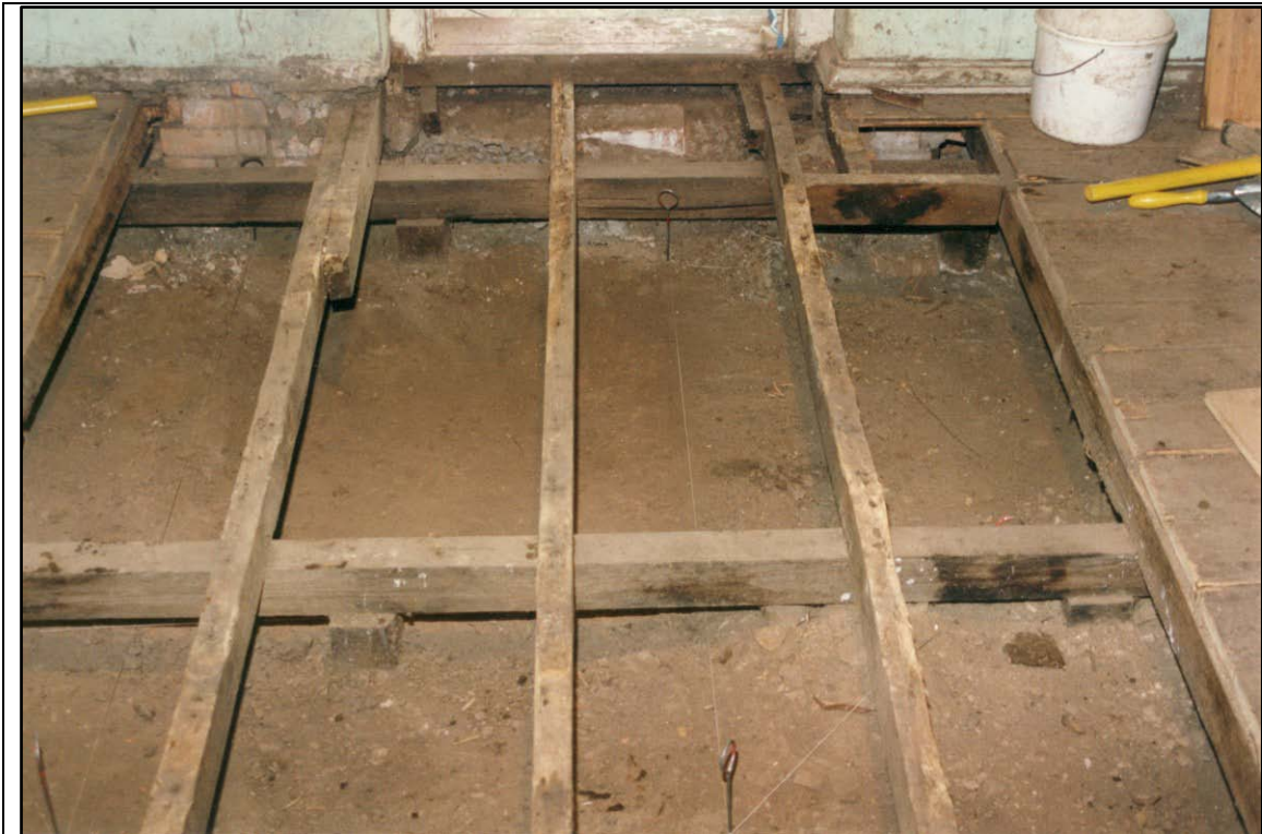
Photograph 59 Trench 5 layout in central room at commencement of excavation marked by string and chaining pins, with front door seen at top of image.
