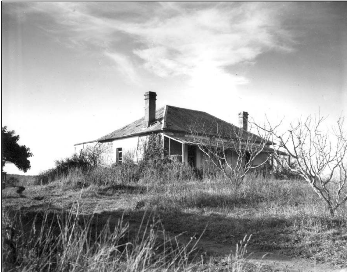
Photograph 5 Shown here in a derelict state is Monckton, built in 1853-55 by Charles Newman from stone and slates. Courtesy Mr Irvine Green as photographed in 1960s. Green reported demolition of this house in 1969.
