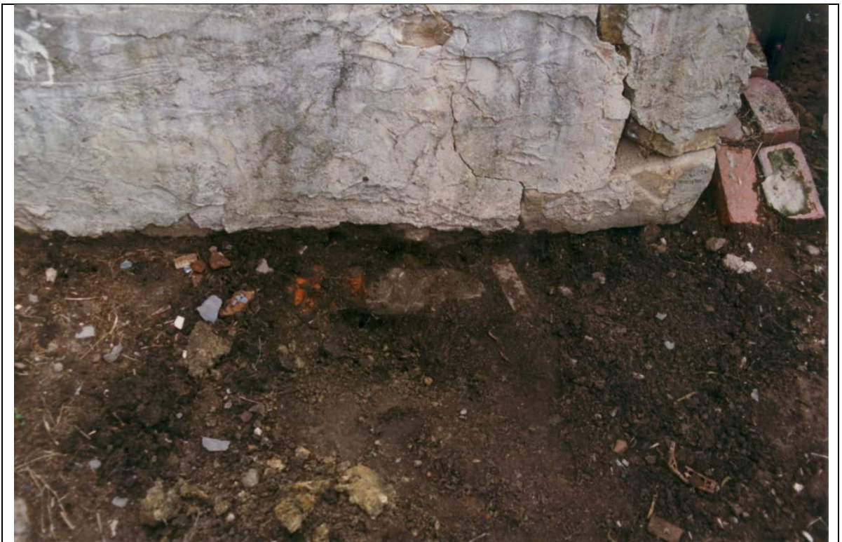
Photograph 54 Seen here is demolition rubble at the eastern edge of the stone tank stand, Trench 3.
