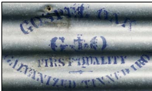
Photograph 38 This brand of Gospel Oak was recorded on galvanized roofing sheets to the kitchen.
