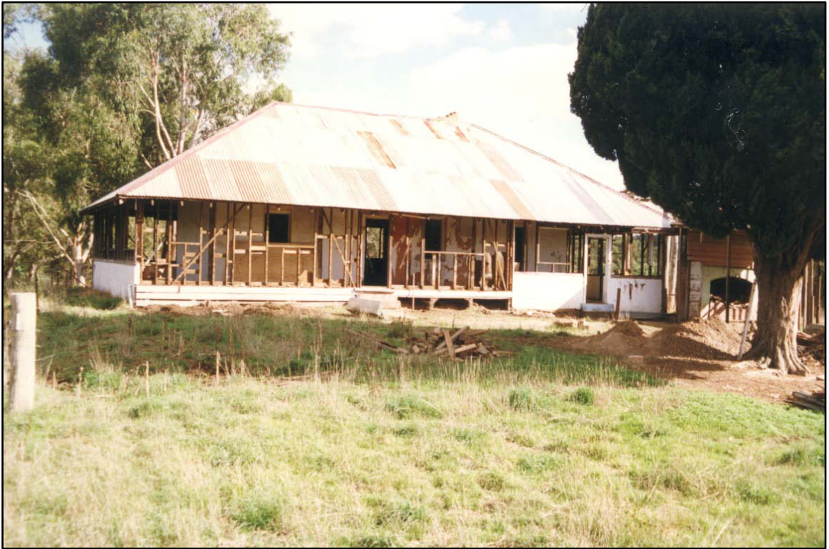
Photograph 8 Rear of Pontville, 1997, during stabilisation program
