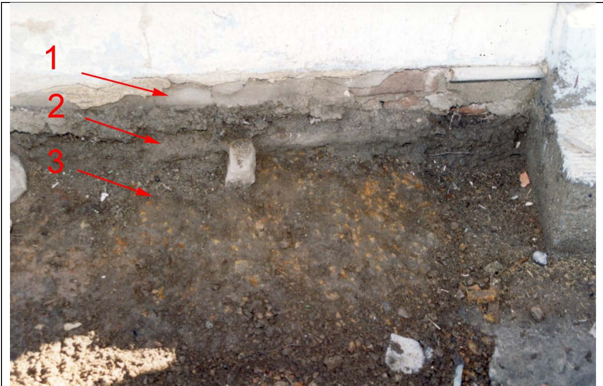
Photograph 56 Seen here are 1) brick footing for the dwarf wall, 2) remnant stone footing of the original verandah, and , 3) orange gravel and clay packing beneath the stone, Trench 4.
