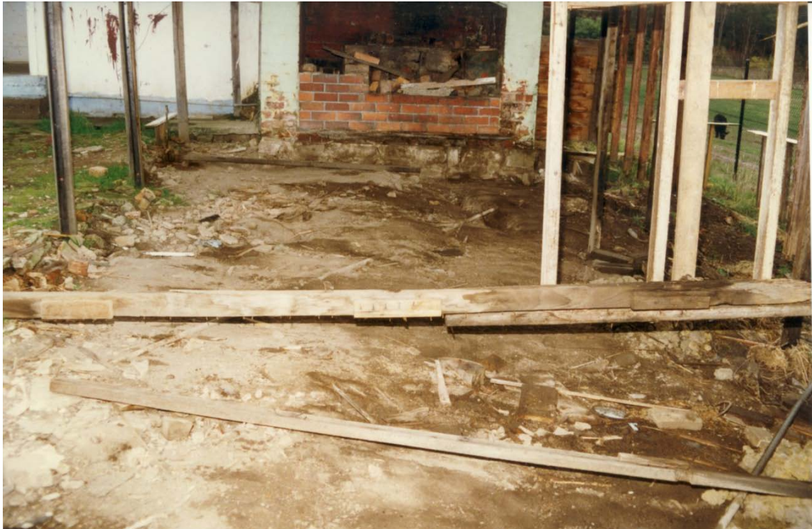
Photograph 36 The detached kitchen in 27 May 1997 at the start of this project.
