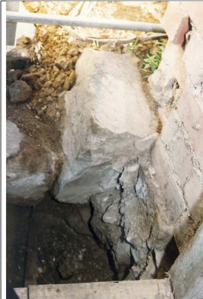
Photograph 47 The thin mortar on the upright footing stone seen here continues behind the brickwork of the chimney, right. Trench 2 at conclusion of excavation.
