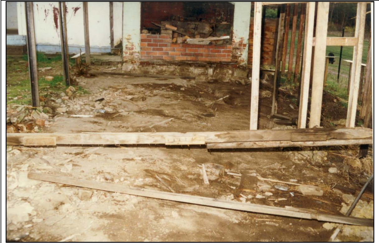
Photograph 41 Trench 1 before excavation commenced in detached kitchen, Pontville
