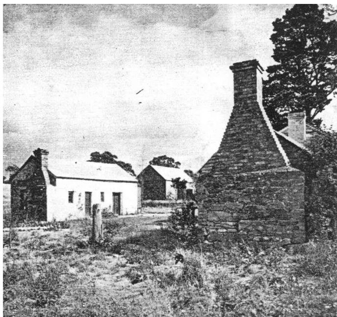
Sweeney's first home at Culla Hill was a 12' x 15' shack of roughly sawn timber palings with a chimney of hand made bricks, still standing and seen on the right of this photo, taken in 1940. In the background are seen the cottage and barn which also belonged to the original homestead
